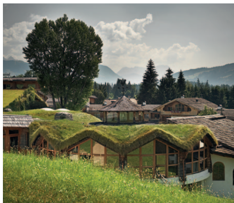
For environmental reasons, all the roofs at the Stanglwirt are made of grass or shingles. Picture: Stanglwirt
